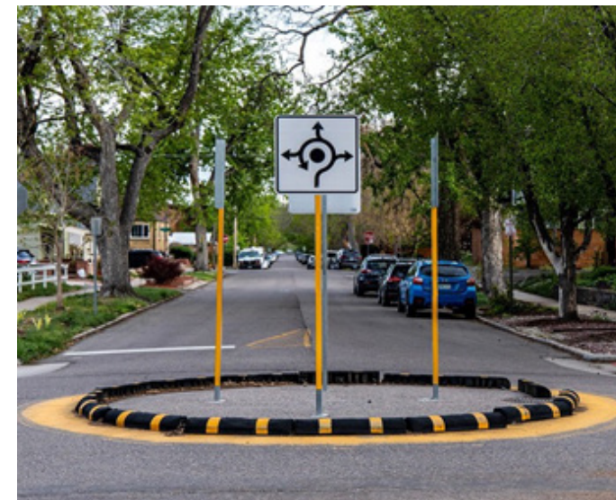
Fig. 21 Mini-Roundabout along Neighborhood Bikeway, Denver
