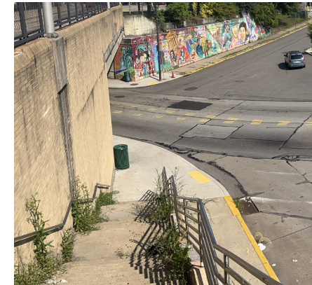
Fig. 28 View North Down the Sawyer Way Stairs
