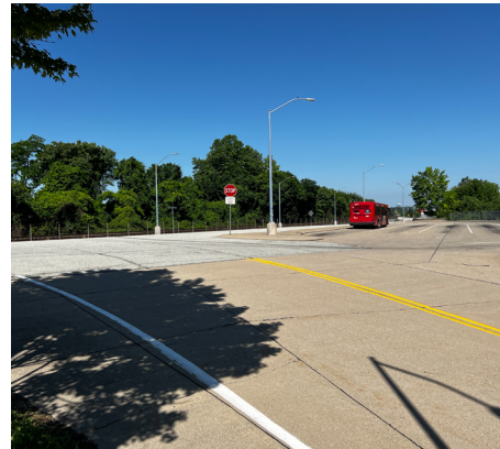
Fig. 32 View of Brushton Avenue Connection to The East Busway
