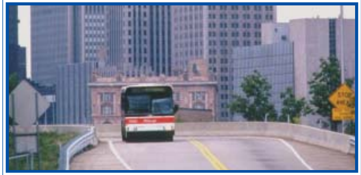
Photo 3.5.2-1 View of the Martin Luther King, Jr. East Busway
