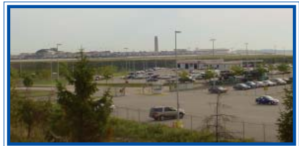
Photo 3.5.3-1 Air Traffic Control Tower and Midfield Terminal at the Pittsburgh International Airport.
