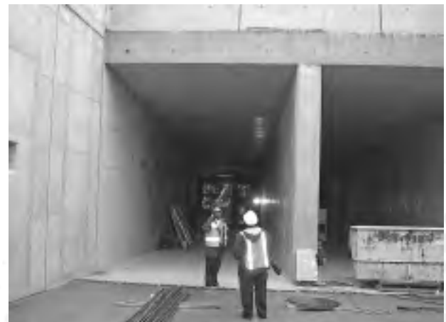
Crews work in the area of the North Side Station portal.
